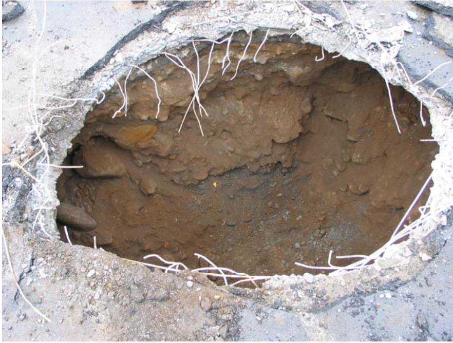
Figure 3. Trench [1]. Upper fills, boulder infill and sea deposits with anthropogenic material.
