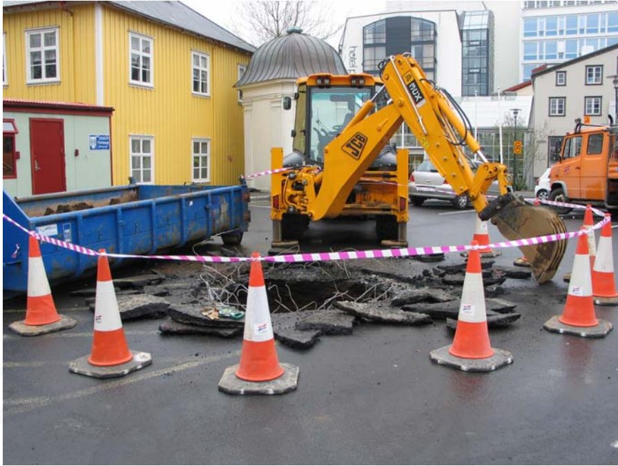
Figure 2. Excavation of trench [1]; 2 nd May 2007.
