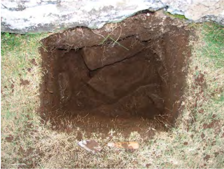
Test Pit 1 Camera direction; Vertical/South
