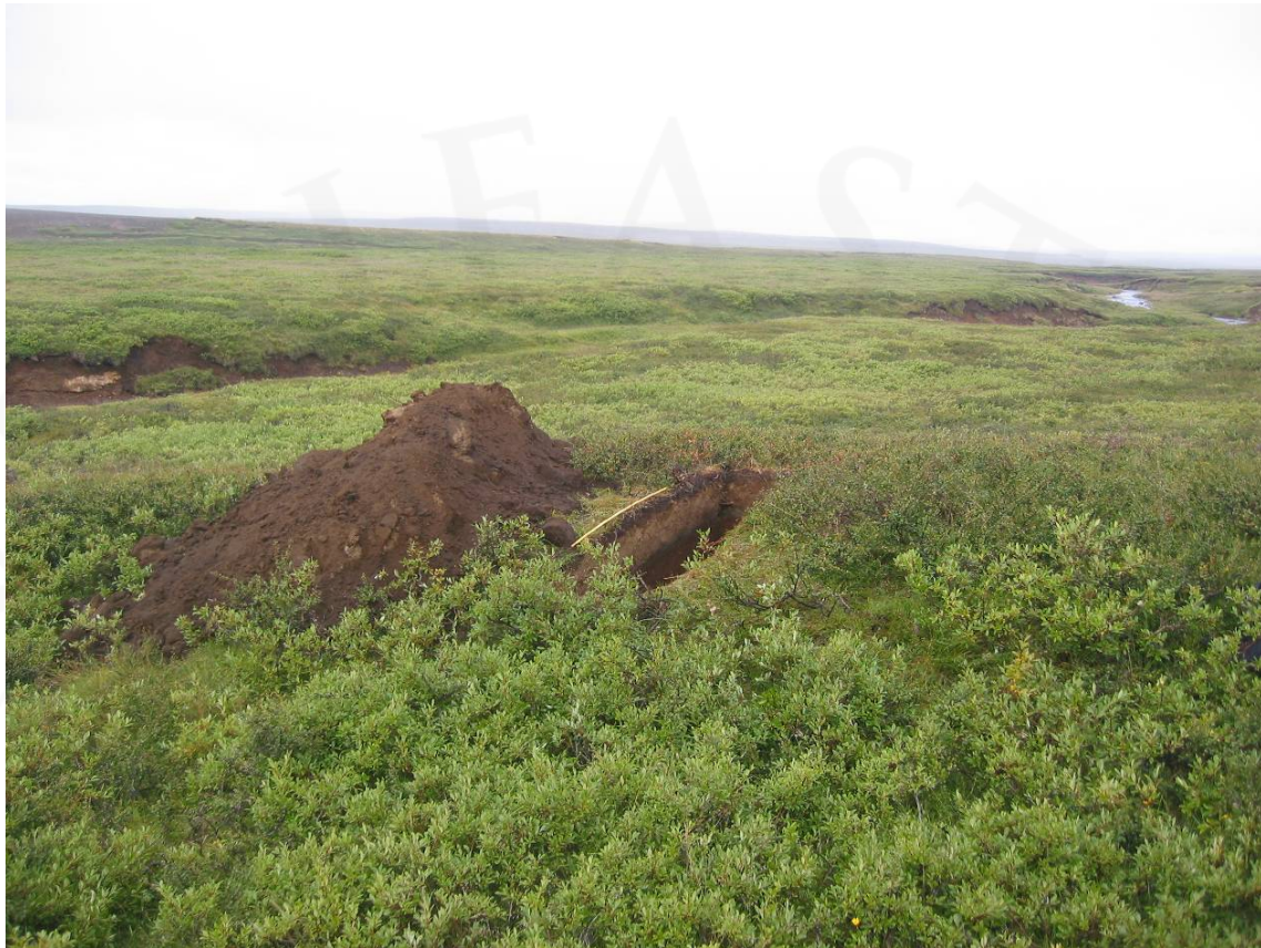
Fig. 33. Trench 1 from the south.
