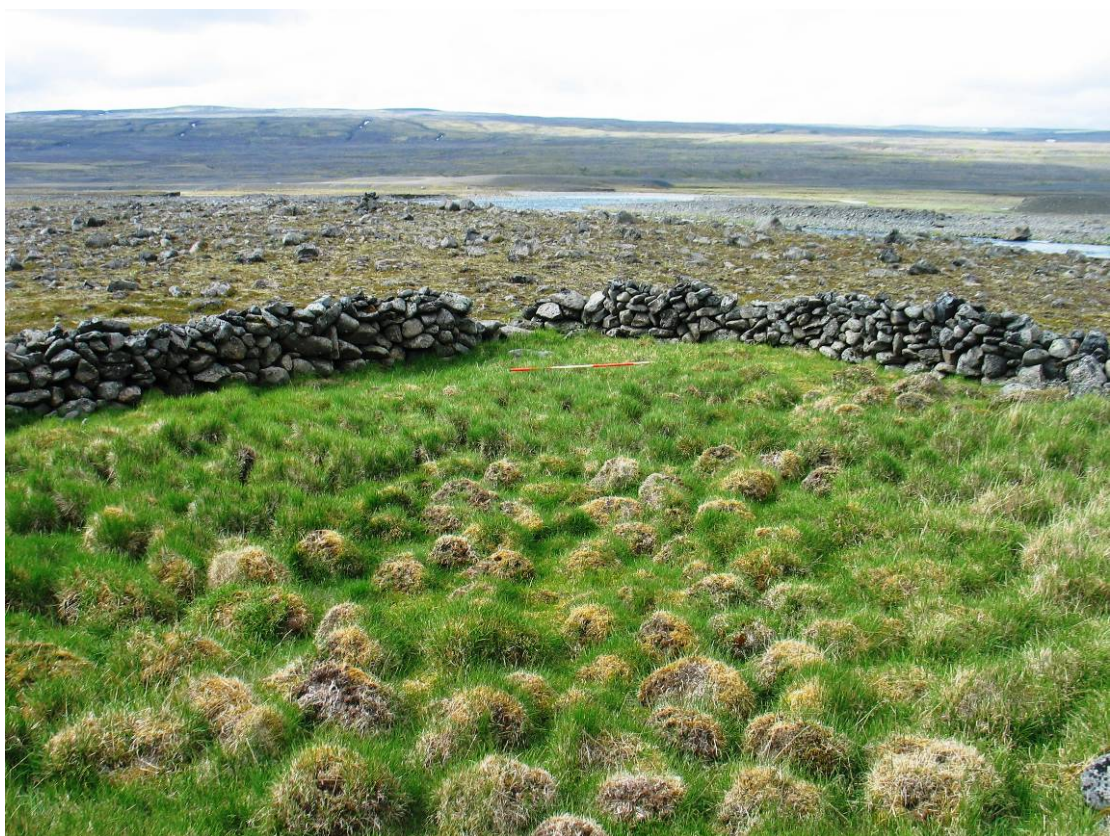
Figure 5. Looking from the inside towards the exterior of the enclosure, looking north (above; Scale 1m); the inside area of the enclosure, at partial collapse in the north-west corner, looking north west (below; Scale 2m).
